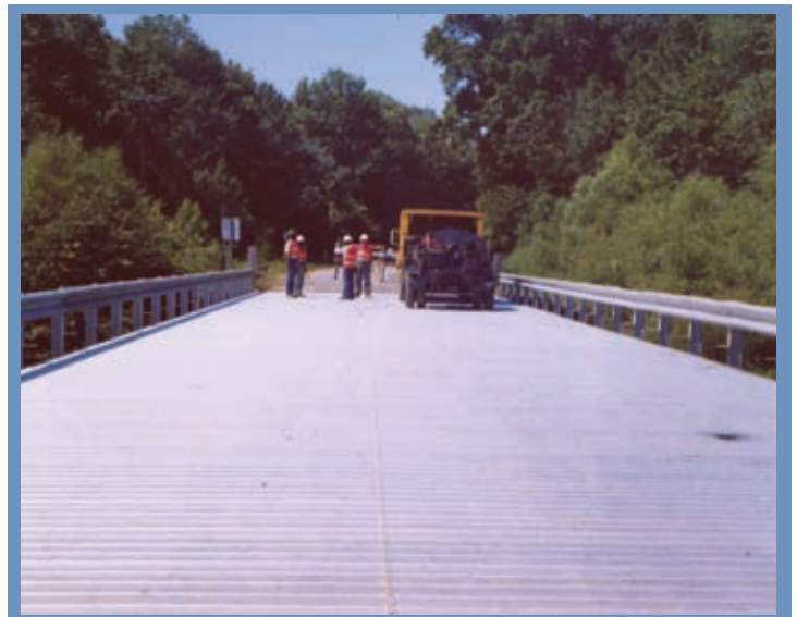
A continuous bridge deck
