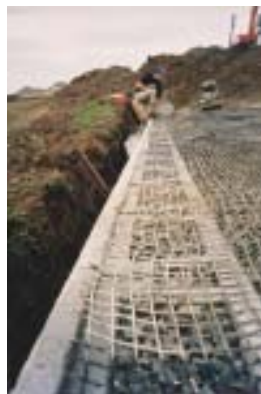
5XT Geogrid and Allan Block working together.
