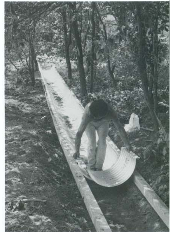
Flanged ditch liner being installed on timber runners.
