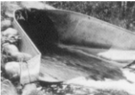
End Section with high outlet velocity helps reduce erosion
